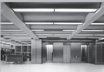
1F Elevator hall
